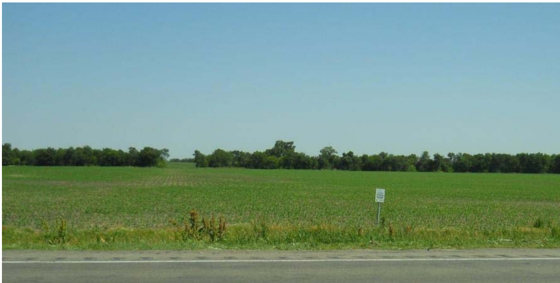
Existing Keystone Oil Pipeline (west of Seward, Nebraska), postconstruction restoration. May 2012. Photo: NDEQ.
