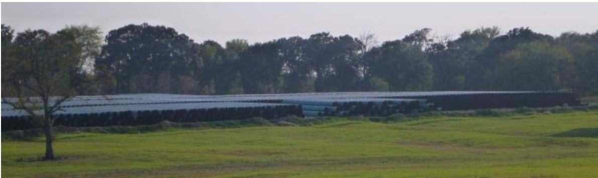
Keystone XL Pipeline Gulf Coast Segment pipe storage yard, Northeast Texas September 2012. Photo: HDR Engineering, Inc.
