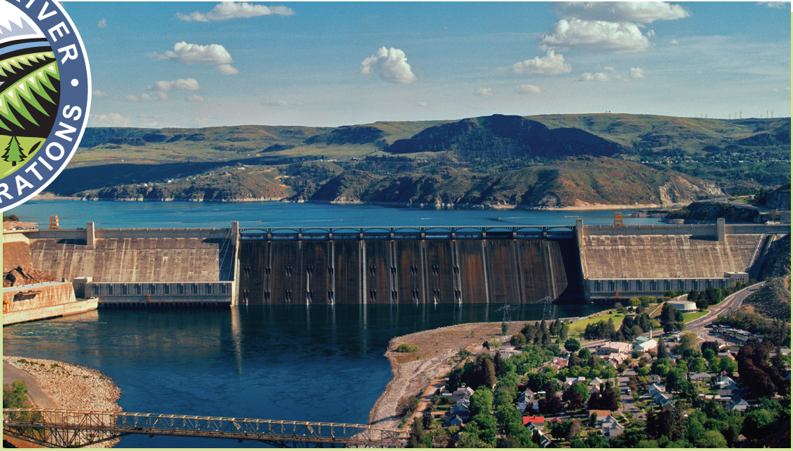
Grand Coulee Dam, Washington
